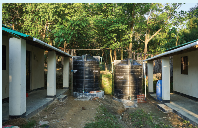
Rain Water Harvesting System
