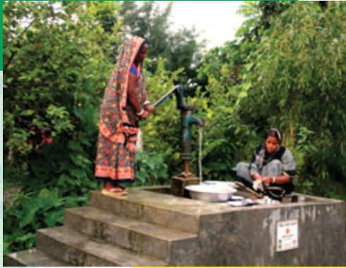
Raised platform tube wells to combat adverse weather events
