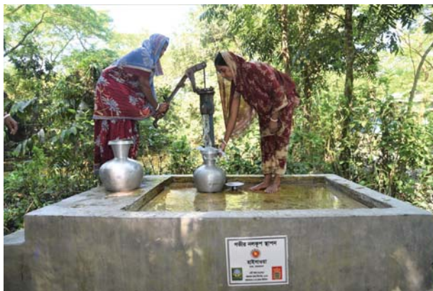
Raised platform tube wells to combat adverse weather events
