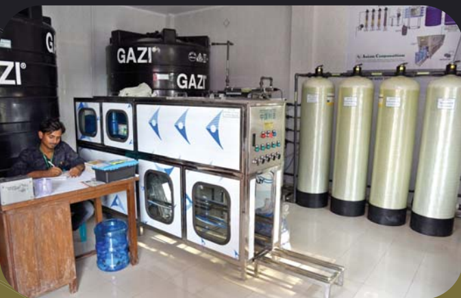
Reverse Osmosis (RO) water treatment plant in Khulna
