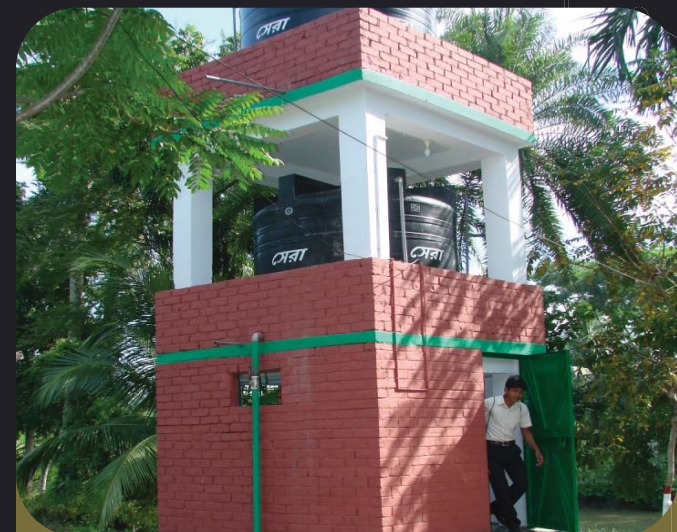
Sky hydrant water purification system in Satkhira
