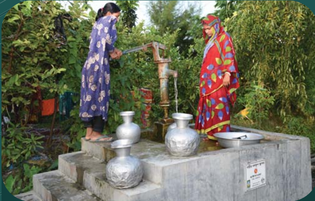
Raised platform tubewells to combat adverse weather events
