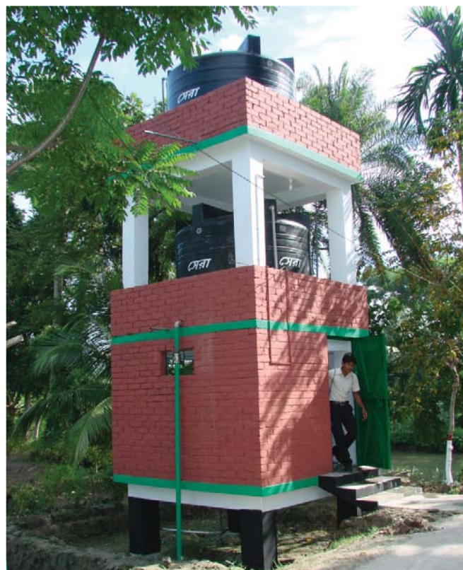
Sky Hydrant Water Purification System at Satkhira
